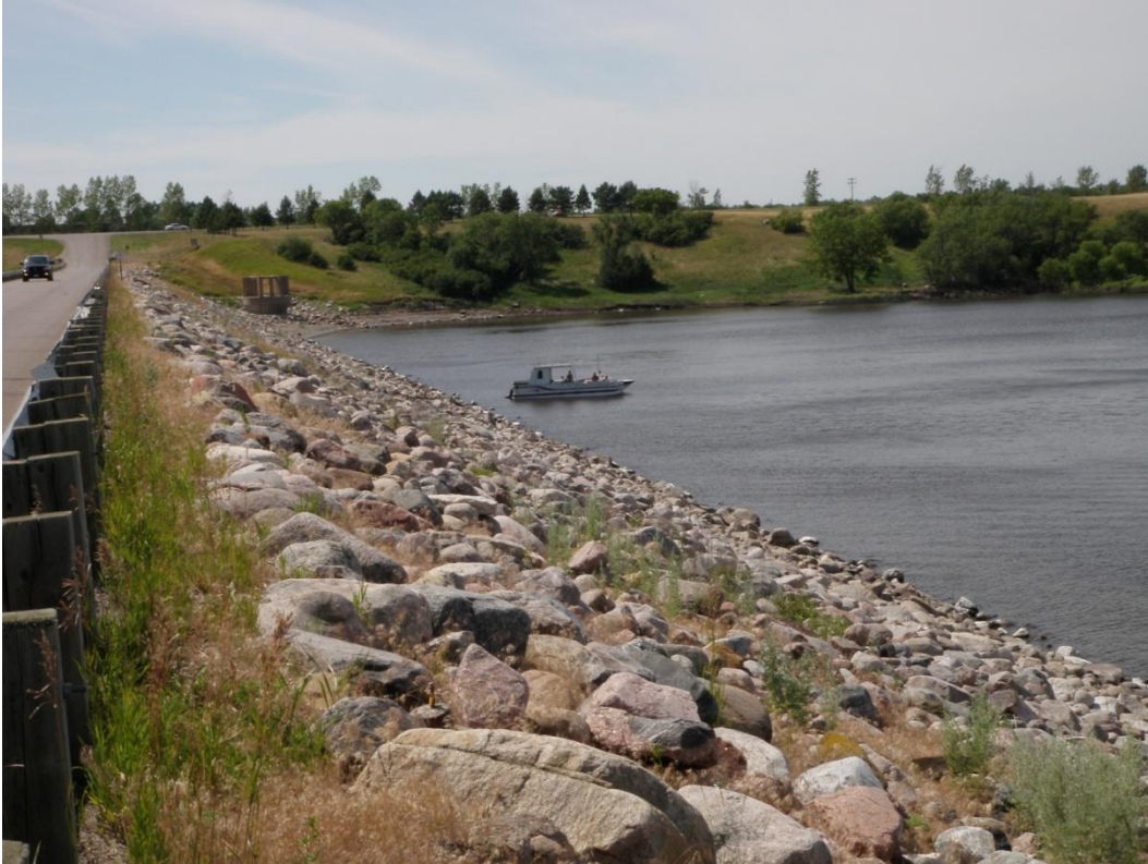
Figure 2 - Top of Jamestown Dam. Looking west towards morning glory spillway.
